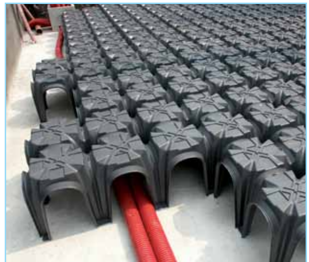
fig. 4) Installation of the MODULO FREEZE
