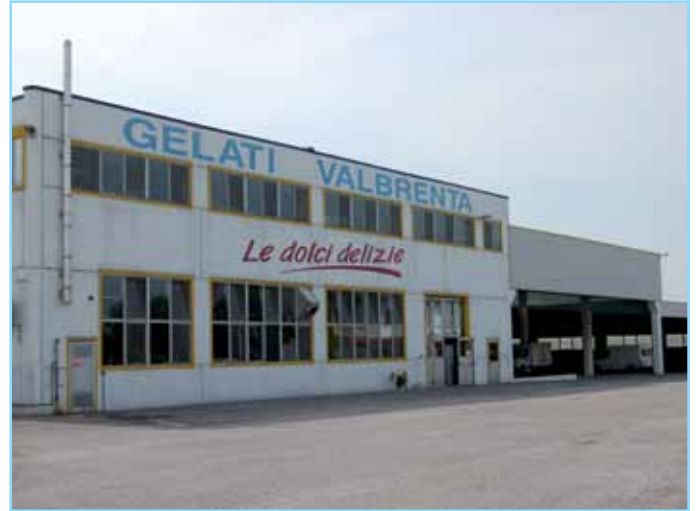
fig. 15) PADOVA • Refrigeration cell 5320 m 2
