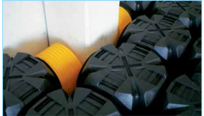
fig. 9) Example of fill-in around a column.
