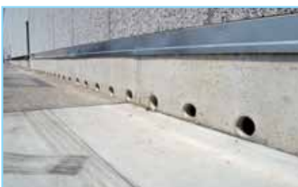
fig. 5) Appropriate external ventilation - Holes approx. every 1 m.
