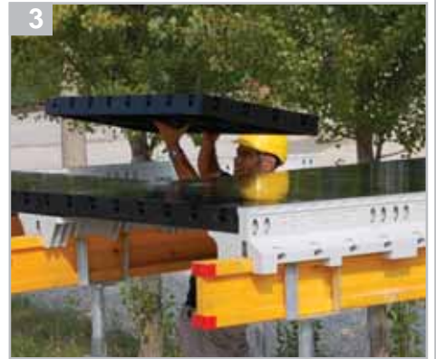
3 Place the GEOPANEL® 120 panel
