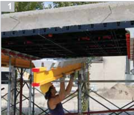
1 Remove the H-beams
