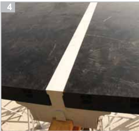
4 Block the panels onto the Y-beams
