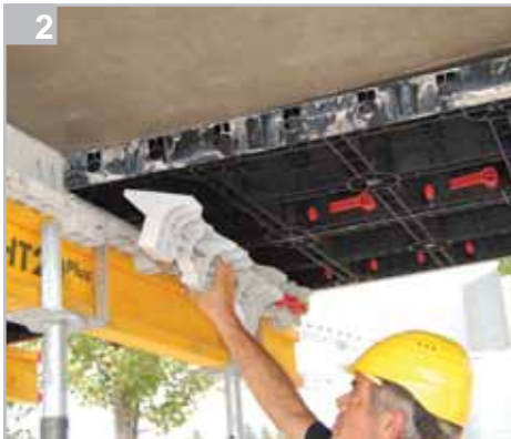
2 Remove the wedges
