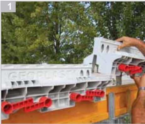
1 Place pre-assembled Y-beam and wedges
