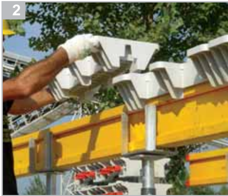
2 Place the H-beam
